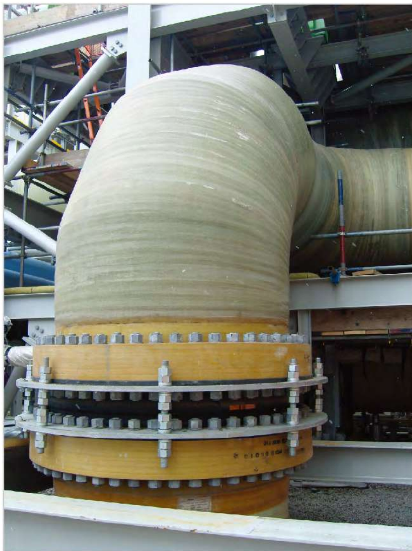
ISLE OF GRAIN POWER PLANT, U.K. EXPANSION JOINT INSTALLATION VIEW
