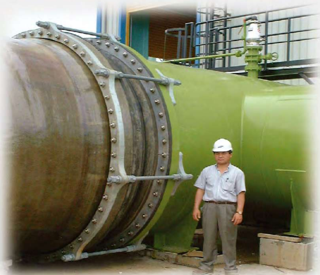
SIEMENS / SERAYA POWER PLANT, SINGAPORE 100 INCH (DN 2500) X 750mmL DOUBLE OPEN ARCH TYPE
