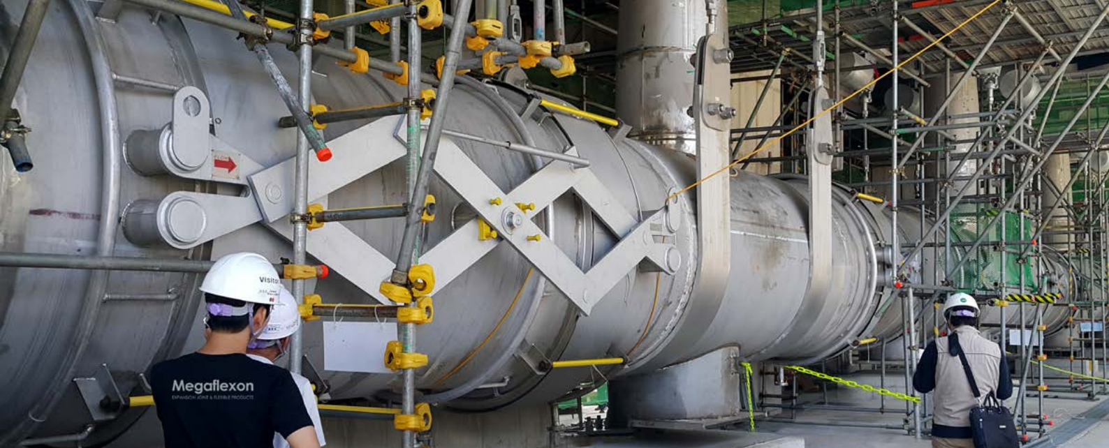
▲ Hot Wall Expansion Joints for PDH Installation View / SK GAS ULSAN PDH PLANT, KOREA
