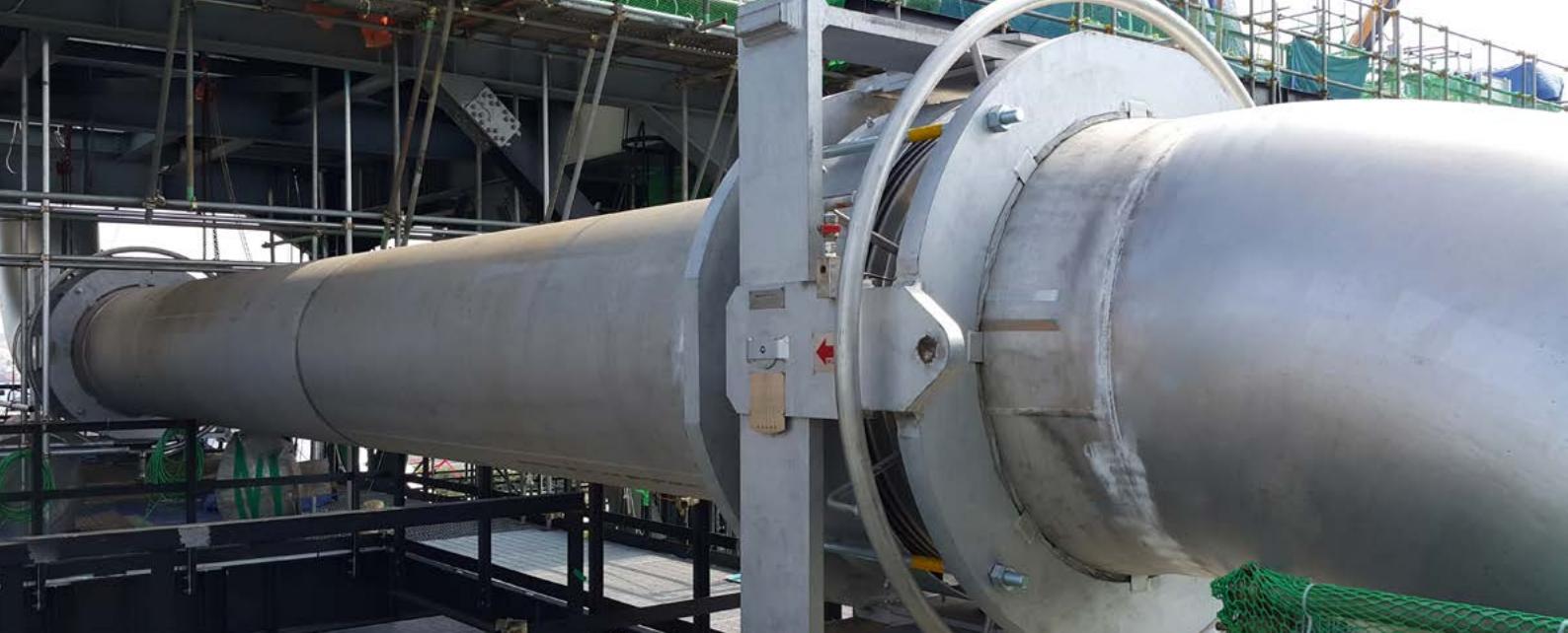
▲ Hot Wall Type Expansion Joints for PDH Installation View / SK GAS ULSAN PDH PLANT, KOREA
